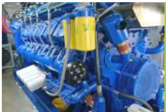
Changsha Huanghua International Airport 1x 1000kW gas engine generator trigenation.
